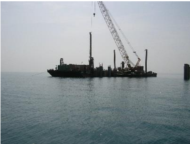
Construction in progress – Abu Dhabi
