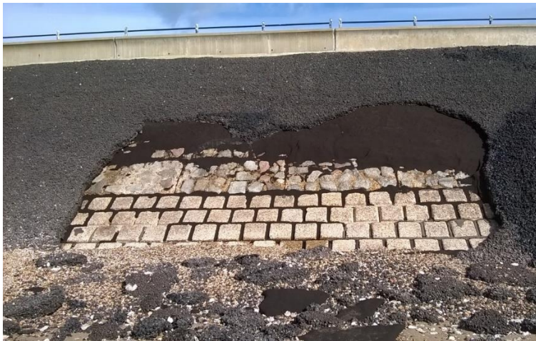
Loss of the open stone revetment revealing the Essex blocks beneath, April 2016
